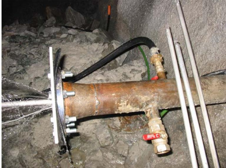
*Figure 3. Picture of the closure system applied at the borehole head to content the water flow.*
